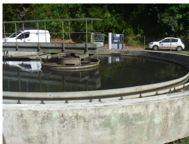
Figure 2.4 - Clarificateur
